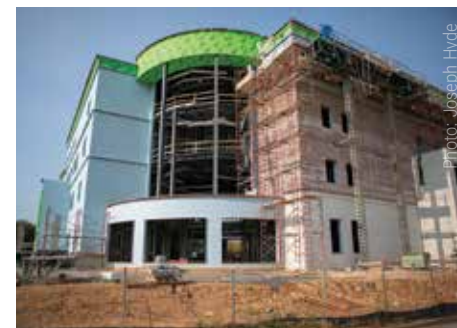
Progress on the Ruth McKee School of Business is well underway.
