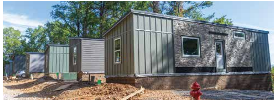
The cottages at the base of White Oak Mountain will embrace the natural beauty of the area once the landscaping and entry decks are completed.
